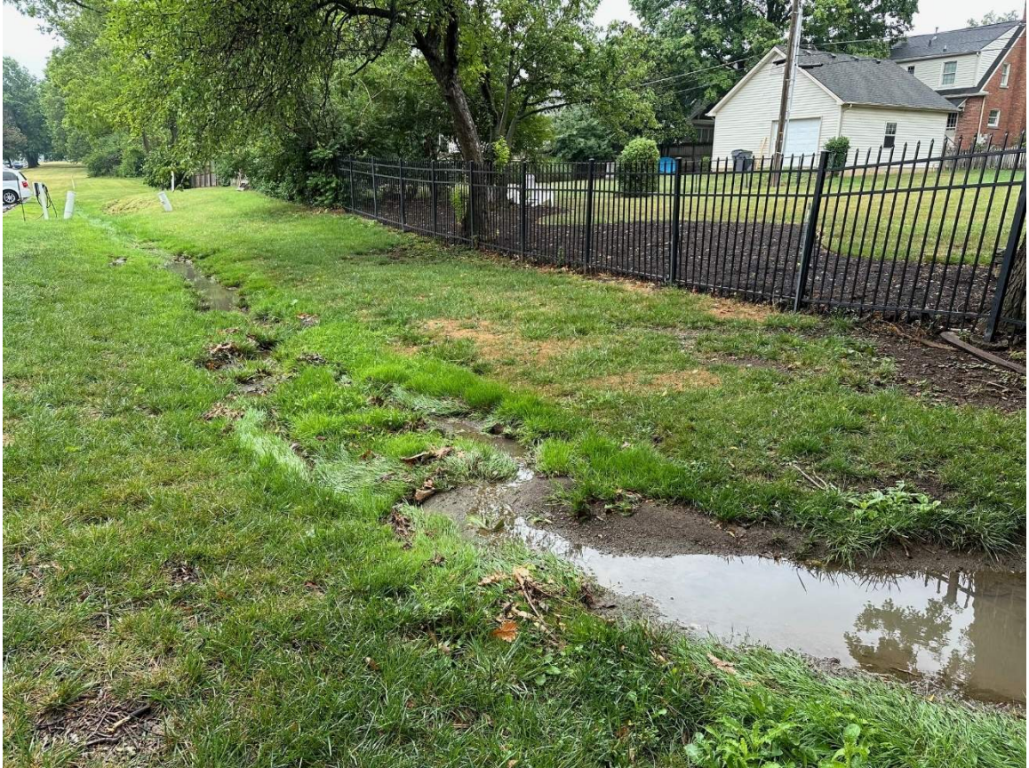
The above image shows the grass swale at the project site. This image was taken on the morning of July 22, 2024 following an estimated rainfall event of approximately 0.17 inches.
