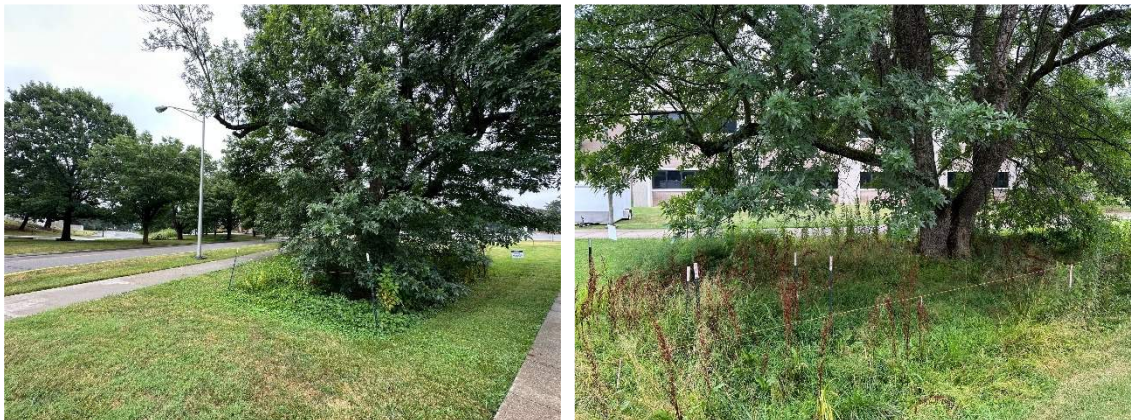
The above images show the location of the spring which has opened by the Oswald Building on Sports Center Drive. The area surrounding the tree pictured has become saturated and poses a potential pedestrian hazard, leading University Grounds staff to construct a temporary barrier around the area.
