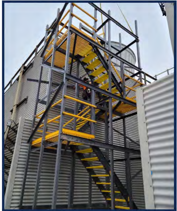
Above: The old wooden stair tower from Med Center Cooling was hoisted down for retirement and replaced with a new and improved fiberglass tower set.
