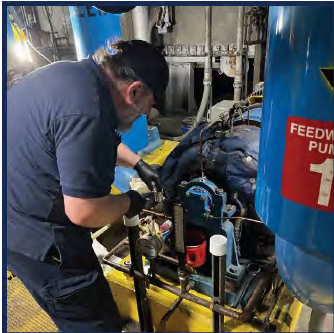
Top L: Scott Barnes and Gary Helton trace an abandoned duct bank outside Pence Hall. Top R: Eric Paullin prepare to perform maintenance on the Stormwater Harvesting System. Bottom L: Eric Connor installs new oiler on feed water pump #1. Bottom R: Steve Booth replaces valve on BFW recirculating line.
