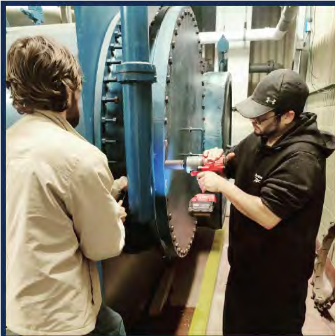
Top L: Ron Mercer, Brian Phippen, and John Nord test relays in sub 3. Top R: Shelby King, Bryan Poe, and Scott Barnes conduct 5-year breaker tests in sub 3. Bottom L: Chris Pelat and Cody Hopewell open chiller #9 condenser. Bottom R: Jack Howard show state inspector boiler #3 mud drum.
