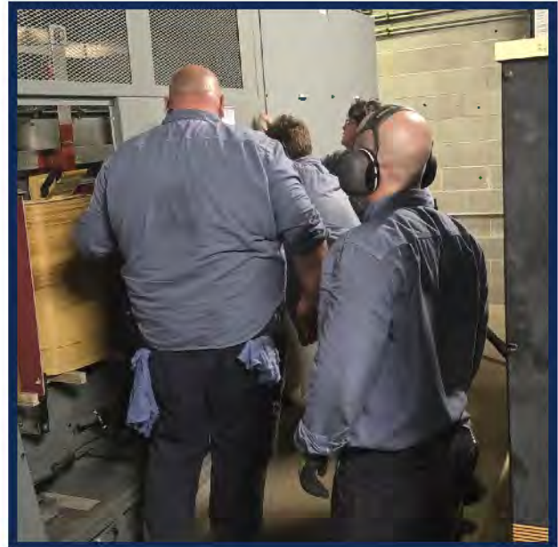
Top: John Nord and Gary Helton coordinate cable cutting in a manhole vault
