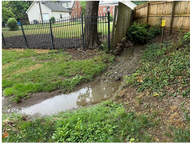
The above images show conditions at the LFUCG outfall from the Montclair neighborhood, located at the head of the grass swale on the Hope Lodge property. Images shown were taken the morning of July 22, 2024.
