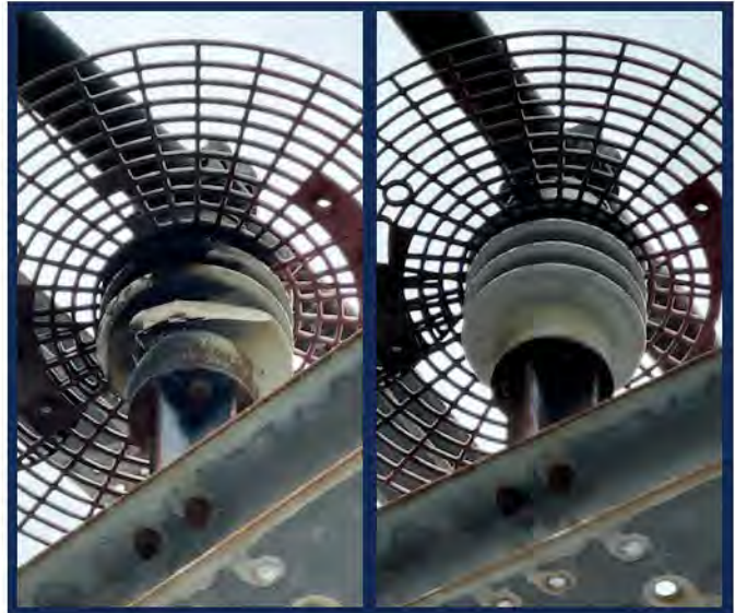
Top L: Robert Hannabach locking out boiler #4 at Med Center. Top R: The High Voltage team prepares PM50 for removal from HEB construction site. Bottom L: KU's relay and control group diagnoses issues with the bus differential CTs at Sub 1 after the squirrel incident. Bottom R: Before/after showing damage to the post insulator by the squirrel and the refurbished replacement insulator in service a few hours later.
