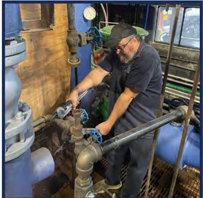
Top L: Scott Barnes and Gary Helton trace an abandoned duct bank outside Pence Hall. Top R: Eric Paullin prepare to perform maintenance on the Stormwater Harvesting System. Bottom L: Eric Connor installs new oiler on feed water pump #1. Bottom R: Steve Booth replaces valve on BFW recirculating line.
