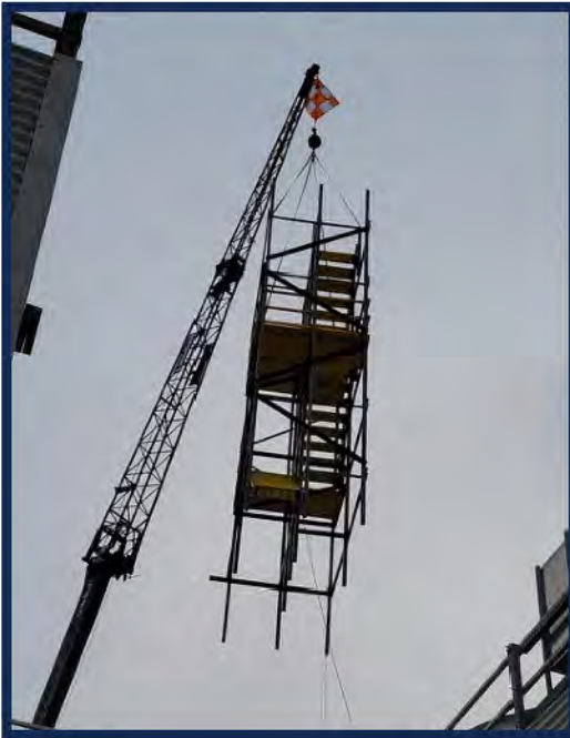
Above: The old wooden stair tower from Med Center Cooling was hoisted down for retirement and replaced with a new and improved fiberglass tower set.
