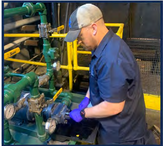
Top L: Britney Ragland receives certificate from Dr. Bob DiPaola for graduating the UK WELD program. Congrats!! Top R: Brian Phippen supervises and conducts annual 12kV switchgear testing at Pav H. Mid R: Chad DeRossitt inspecting rotor and spindle on fuel oil pumps. Bot: Ron Mercer leads the High Voltage team in substation breaker relay training.
