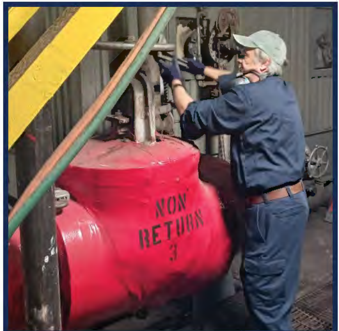
Top L: Duct bank installation continues for the HEB project. Top R: Gary Helton operates a high voltage switch at electrical vault E122 while Marcelo Campos assists. Bottom L: Jack Baysore doing some housekeeping around the Med Center coal bunker. Bottom R: Joe Cafego opening non-return valve on MC Boiler #3.
