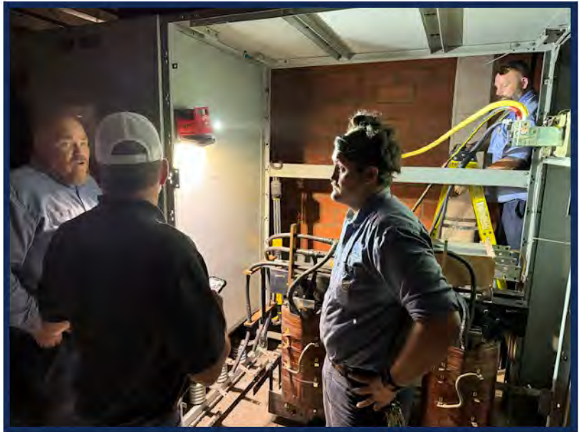
Top: John Nord and Gary Helton work out a plan for moving the Animal Pathology transformer with American Industrial Contractors while Zach Saunier of the Electric Shop hooks up the Emergency Generator.
