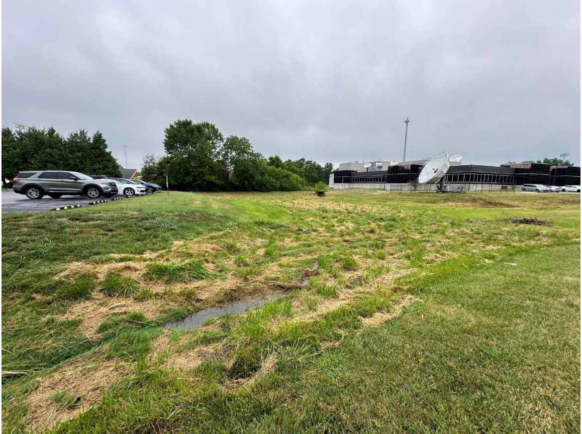
The above image shows the grass swale and basin at the project site. This image was taken on the morning of July 22, 2024 following an estimated rainfall event of approximately 0.17 inches.
