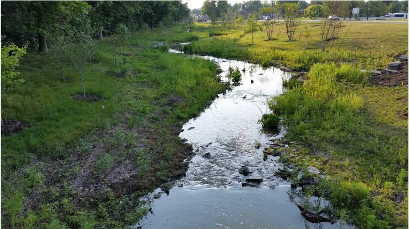
After filling and grading the floodplain, sowing seed, planting new trees, and waiting four months, Big Elm Fork looks more like a natural stream and can spread out over a wider floodplain during storms.
