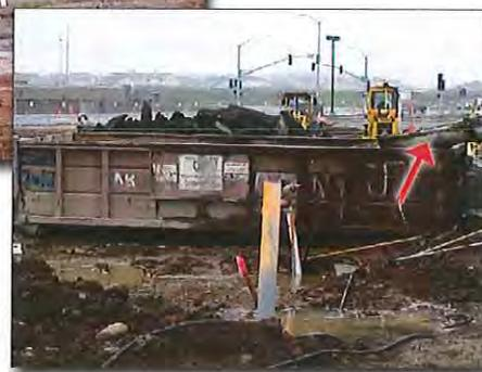
**Figure 2.** Chute washwater leaking from a roll-off bin being used as a washout container
