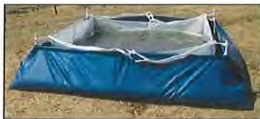
Figure 11. Vinyl washout pit with filter bag
