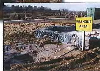
Figure 10. Leaking washout pit that has not been well maintained
