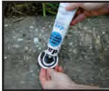
Apply adhesive to the back of the marker as shown. Start 1/8" in from the outside edge, applying an even bead around the entire edge, and then work to the center.
