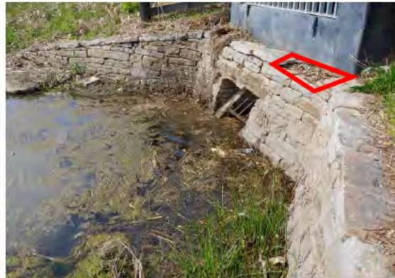
***Lower Basin (3.1): The outfall inlet of the basin was cleared of obstructions to ensure proper flow. Missing capstone rock (outlined above right) from basin outlet.***
