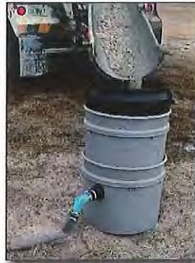
**Figure 3.** Concrete washout filter
