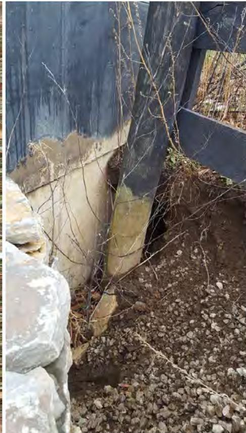
***Upper Basin (3.5): There are two growing cavities around the basins outlet structure.***
