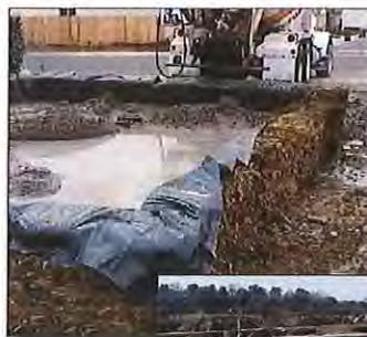
Figure 9. Hay bale and plastic washout pit
