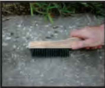
Clean application surface with wire brush. Surface must be clean, dry, and free of any loose debris. *The presence of any foreign material (paint, oil, etc.) may affect adhesion.*
