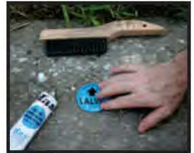
Place the marker on the application surface. Push down HARD with a twisting motion, forcing adhesive out from the edge. It is important that the entire edge of the marker is sealed to the application surface.
