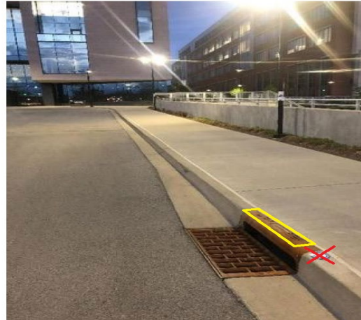
Figure 9: Storm drains with a permanent identifier (i.e. cast/lettered with “No Dumping, Drains to Stream/River”) should not be marked, they should be designated as Yes-Permanently Cast/Lettered
