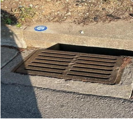
Figure 7: Drains that are not permanently cast/lettered and were marked as part of this survey, should be designated as Yes-Temporary Marker
