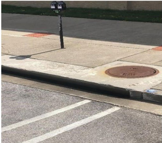
Figure 6: Drains that are not permanently cast/lettered and were marked as part of this survey, should be designated as Yes-Temporary Marker
