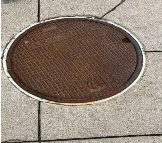
Figure 5: Solid lid manholes are not storm drains. They should not be marked as part of this program.
