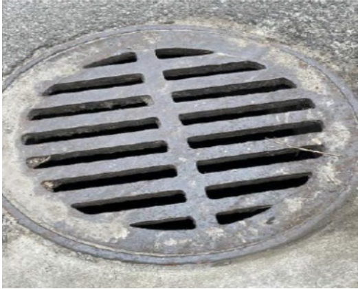
Figure 4: Drains in roadways without adjacent curbing or other hazardous areas should not be marked. They should be designated as No-Marker Not Required .
