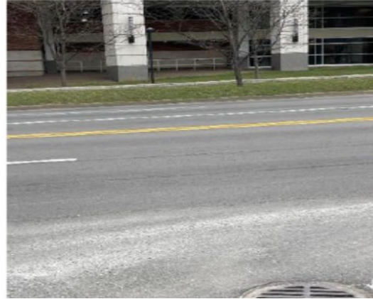
Figure 4: Drains in roadways without adjacent curbing or other hazardous areas should not be marked. They should be designated as No-Marker Not Required .
