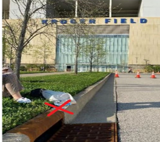
Figure 8: Storm drains with a permanent identifier (i.e. cast/lettered with “No Dumping, Drains to Stream/River”) should not be marked, they should be designated as Yes-Permanently Cast/Lettered
