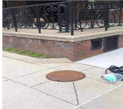
Figure 5: Solid lid manholes are not storm drains. They should not be marked as part of this program.
