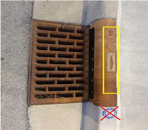
Figure 9: Storm drains with a permanent identifier (i.e. cast/lettered with “No Dumping, Drains to Stream/River”) should not be marked, they should be designated as Yes-Permanently Cast/Lettered
