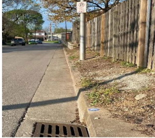
Figure 7: Drains that are not permanently cast/lettered and were marked as part of this survey, should be designated as Yes-Temporary Marker
