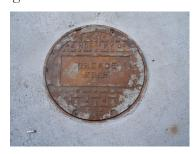
External grease trap: These are located outdoors and should be pumped/cleaned by a grease hauler at least every six months or as required by your permit.
