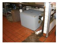
Internal grease trap: These are located near the sink area and can be above ground or in the floor. These should be cleaned at least once a week or as often as your permit requires.
